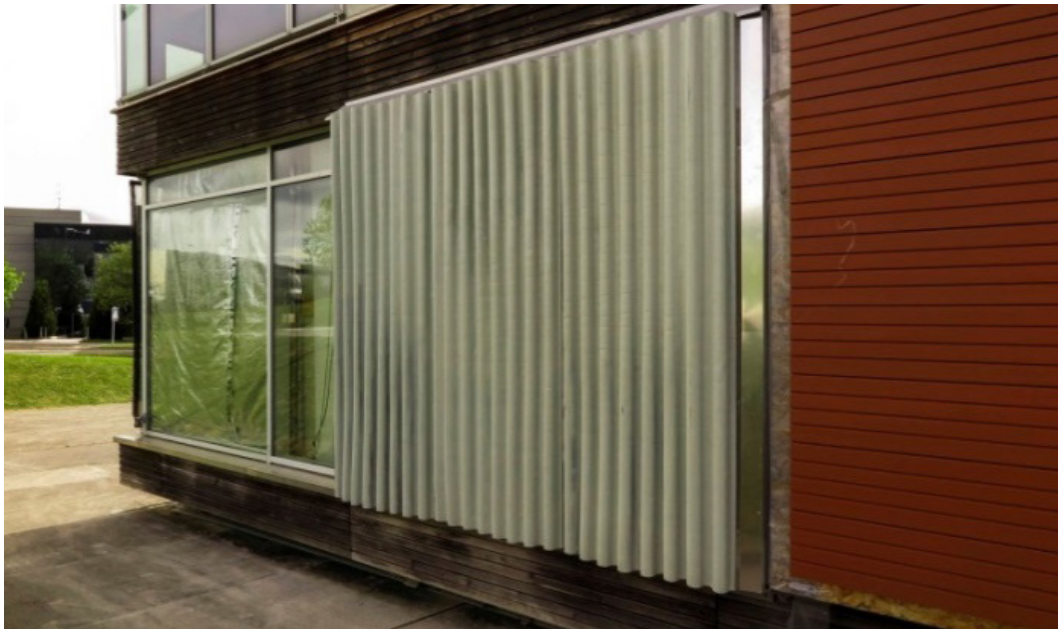
FIG. 6 Multilayer façade installed in Kubik test cell
