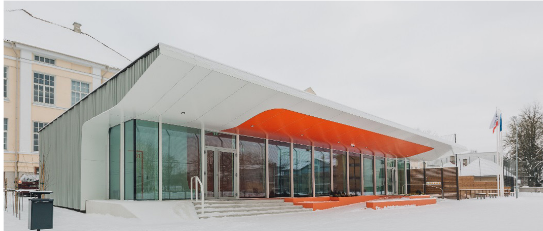
FIG. 8 External view of the Tartu demo building. The front curtain wall was developed through the Osirys project like the rest of the façades (which use the multilayer façade solution). The partitions inside the building also use the Osirys developments.
